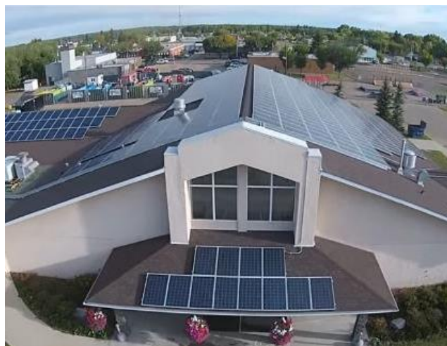
Devon Community Centre 100 kW
