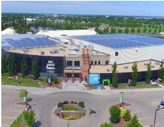
Leduc Recreation Centre 1,111 kW
