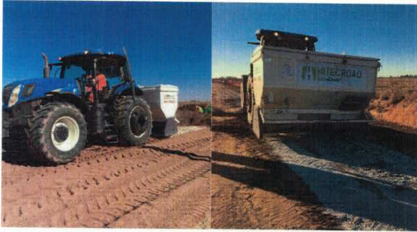
c. Spreading of the exactly amount of cement per square meter ( m^2 )
