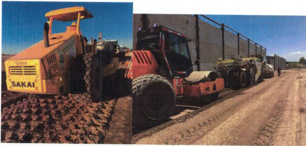
f. Fine leveling by using a grader
