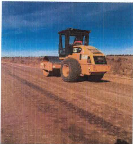
h. Curing after final compaction (min. 3 days)
