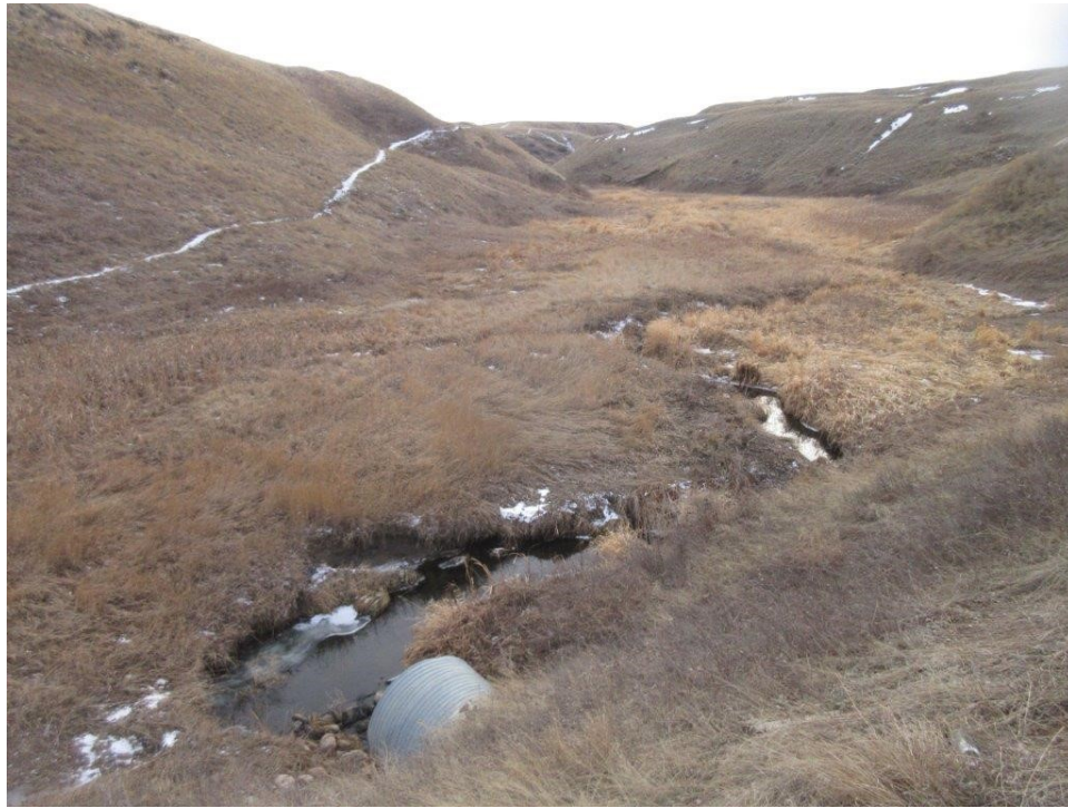
3. Channel alignment looking U/S south. Channel is poorly aligned to culvert causing localized erosion of the U/S banks.
