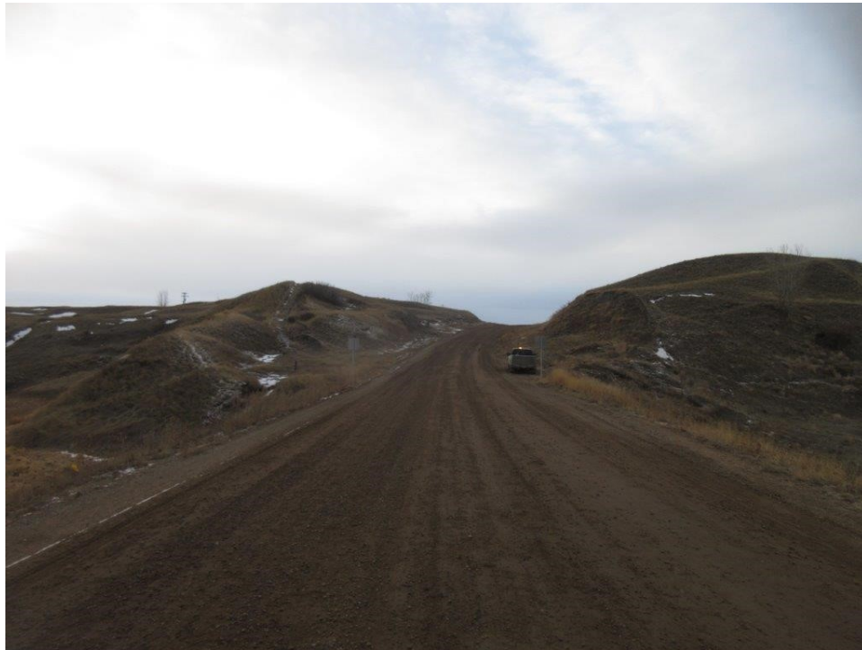
1. Road alignment looking west on waste transfer road in Taber.
