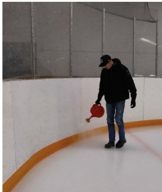
Photo 4: Current process of "flooding" the corners of the ice where the Zamboni cannot reach.
