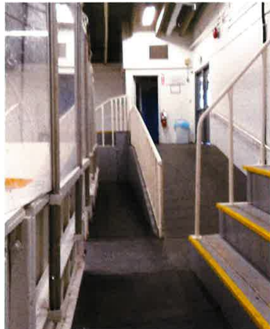
Photo 2: Access Ramp at east end of rink.
