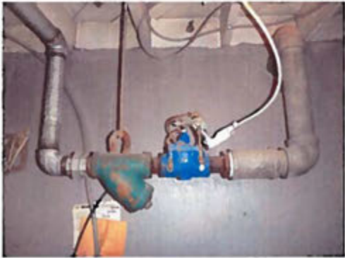
50MM CONTROL VALVE AND STRAINER
