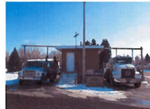
BULK FILL STATION LOOKING SOUTH
