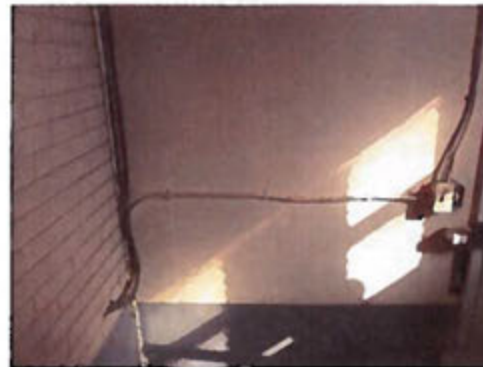
REAR STAIRWELL TO BASEMENT
