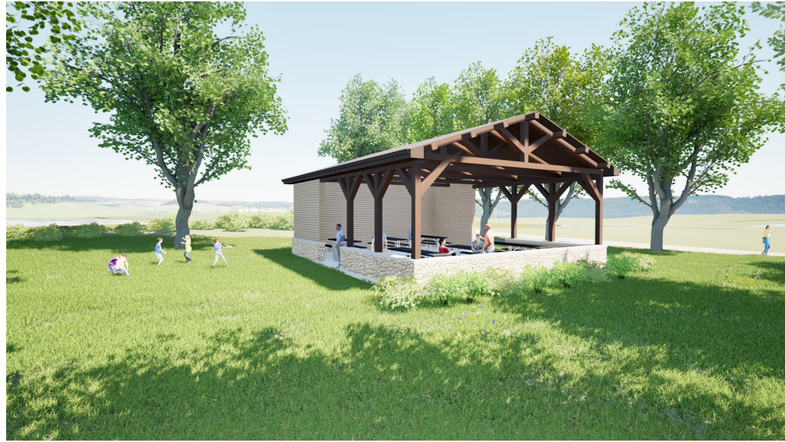
OPTION 5 - WOOD CONSTRUCTION - PONY WALL - REDUCED AREA
