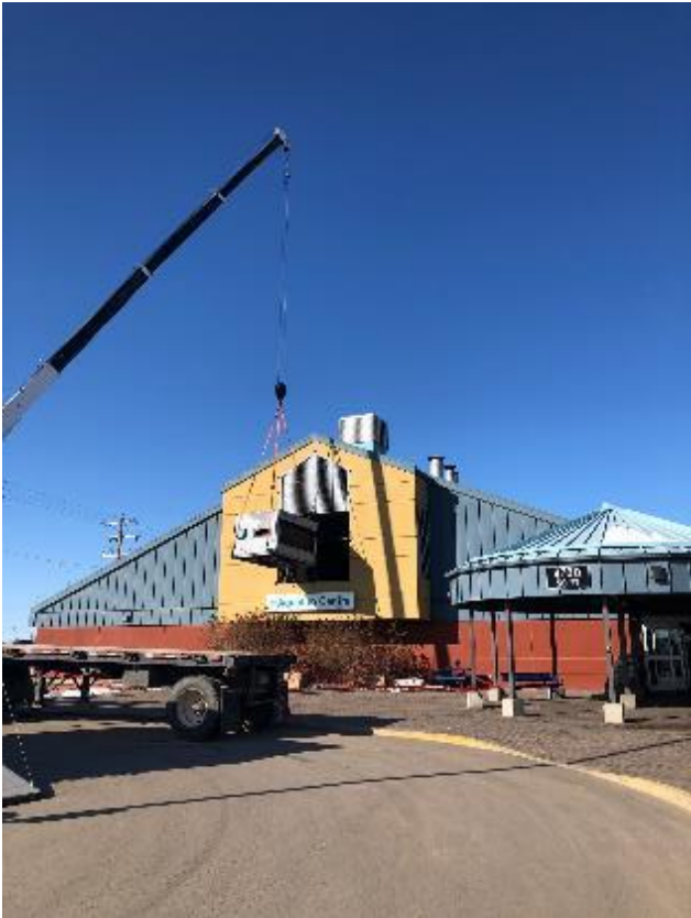
ECM 65: Replace heat exchanger on AHU
