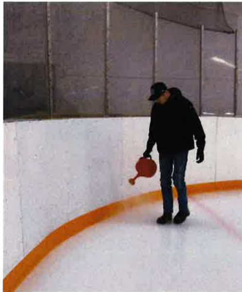
Photo 4: Current process of "flooding" the corners of the ice where the Zamboni cannot reach.
