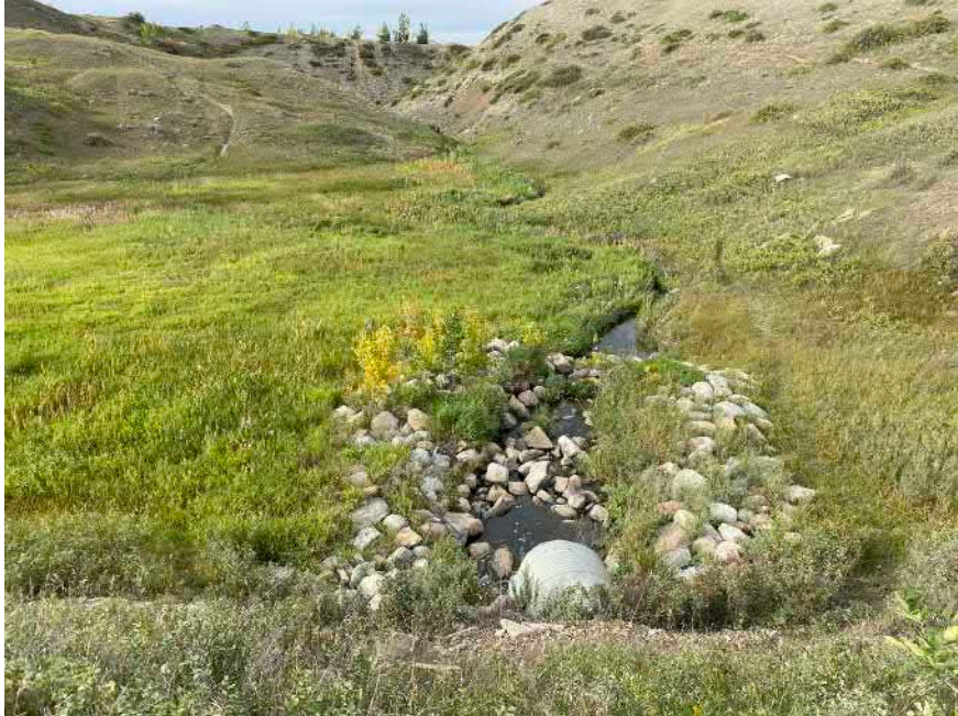
Figure 4. North side of Culvert BF 80500
