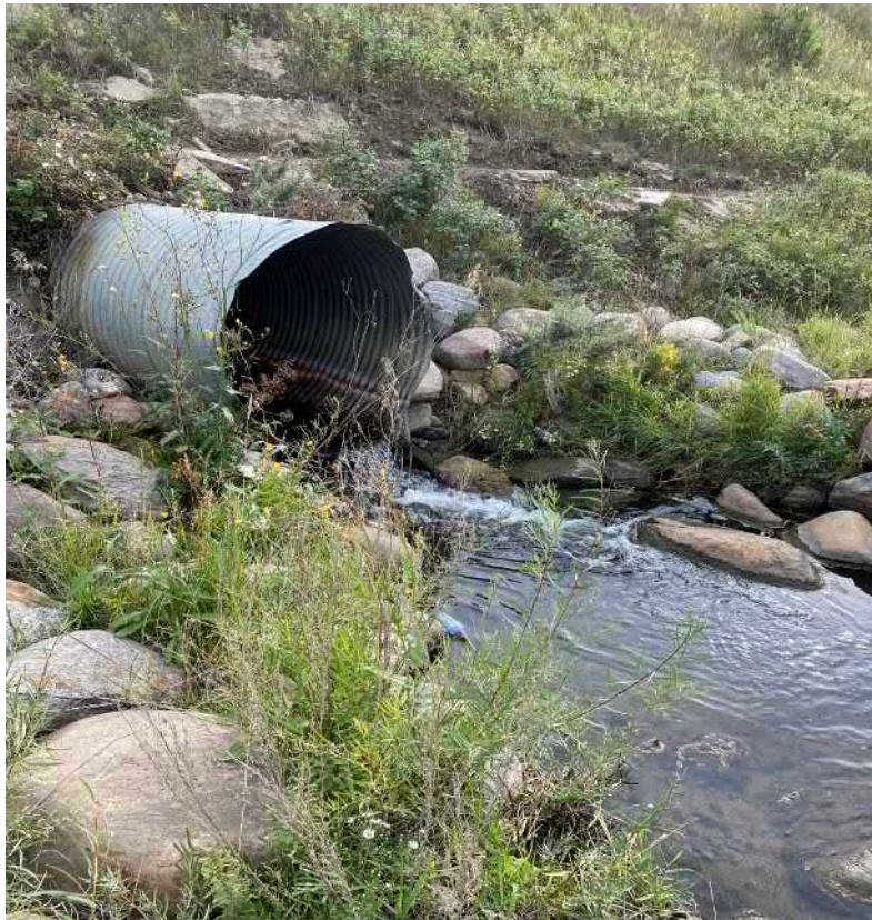
Figure 5. North side of Culvert BF 80500.
