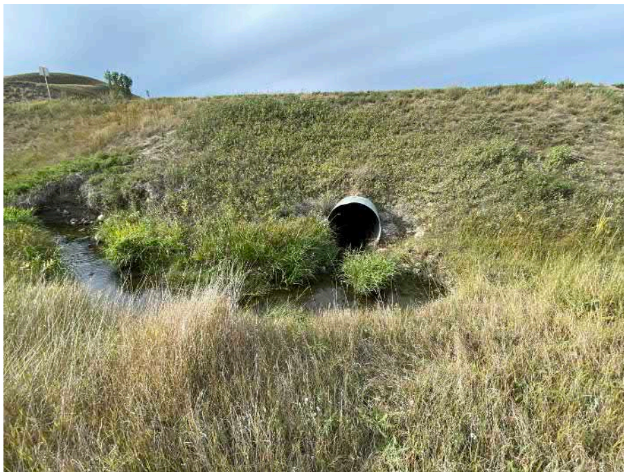
Figure 3. South side of culvert BF 80500
