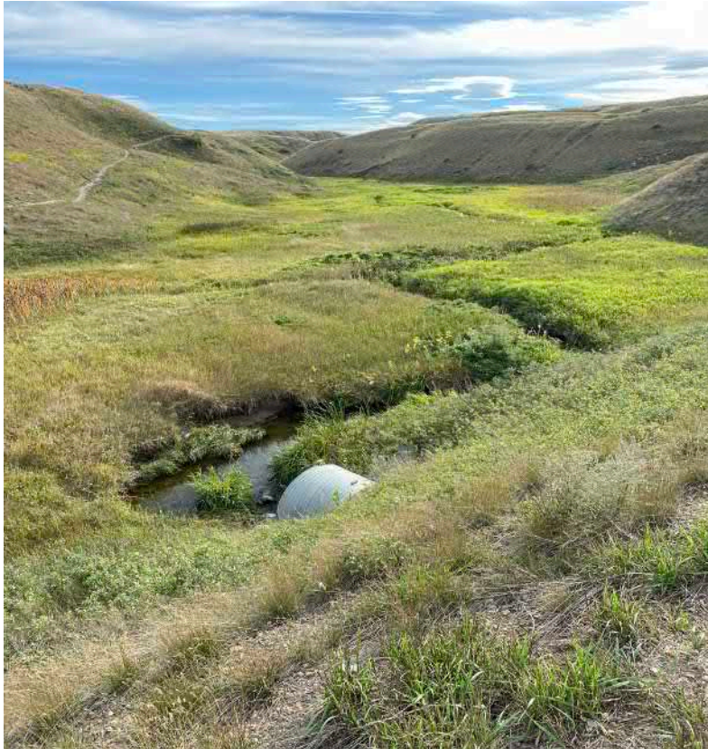
Figure 2. Culvert BF 80500, view south.
