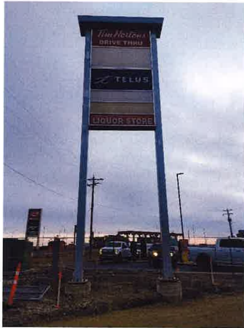
PHOTO 1 – OVERALL EXISTING SIGN (LOOKING EAST)
