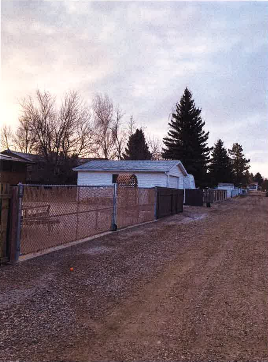
This is the garage they would remove and the area where the new garage would be built.
