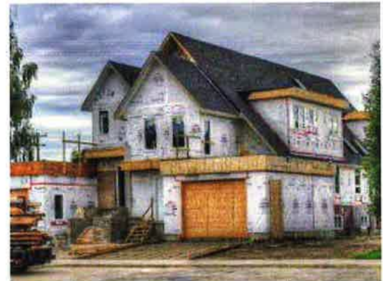
New residential construction
